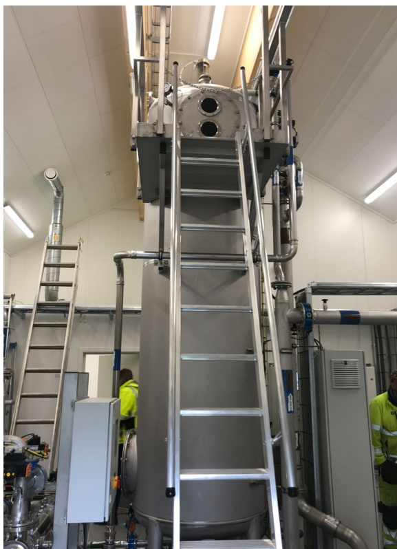
Figur 23: Ozon- Biofilter
